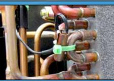
A sensor placed on the outdoor coil will stop the compressor operation if excessive refrigerant temperatures are detected, prolonging the compressor life.
