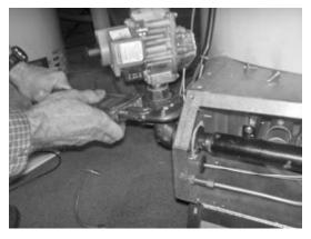
Step 5: Disconnect and Remove Gas Valve
