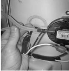
Check pressure switch tubing to the pressure switch. Make sure tubing does not have kinks, holes, condensate, or dirt blocking air pressure to the switch. The tubing to the blower tap attaches to the - (minus) tap on the pressure switch.
