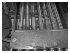
Step 14: Slide out burner assembly
