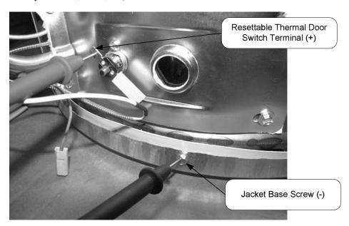
Normal thermopile operation will be between 350 mV - 850 mV. If reading is less than 350 mV, replacement of pilot assembly is recommended following SERVICE PROCEDURE RG-III.
