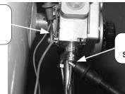
Alligator clip to copper sheath of thermocouple
