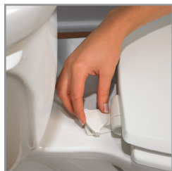
TWIST HINGES TO UNLOCK
