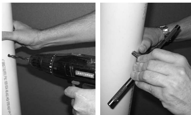
Figure 9.1: Drill and Tap Combustion Test Port
