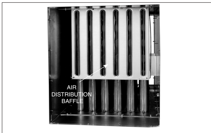
Figure 4.2 Air Distribution Baffle Location
