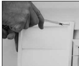
**3** Push the hood into the opening and then attach the hood to the outside wall with mounting screws. Repeat the installation procedure for both the supply and exhaust hoods.
