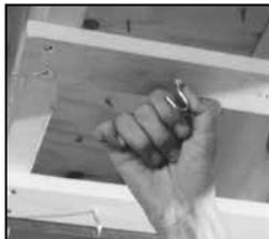
1. Place fastening hooks on the strapping board or the floor joists.
