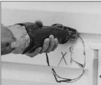
**1** Using the duct connection of the outside hood, outline the intake & exhaust holes to be cut. The holes should be slightly larger than the duct connection to allow for the thickness of the insulated flexible duct. Cut a hole for both the intake and exhaust hoods.
