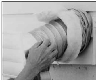
**2** Pull the insulated flexible duct through the opening until it is well extended and straight. Slide the duct's inner vinyl sleeve over the hood duct connection and secure. Pull the insulation over the duct and pull the vapor barrier over the sleeve. Secure with appropriate tape or sealant.
