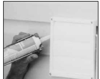
**4** Using a caulking gun, seal around both hoods to prevent any leaks.
