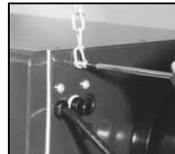
2. Attach a hanging chain to each corner of unit using provided screws and washers.
