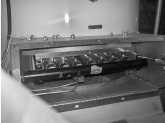
Step 7: Remove manifold bracket screws
