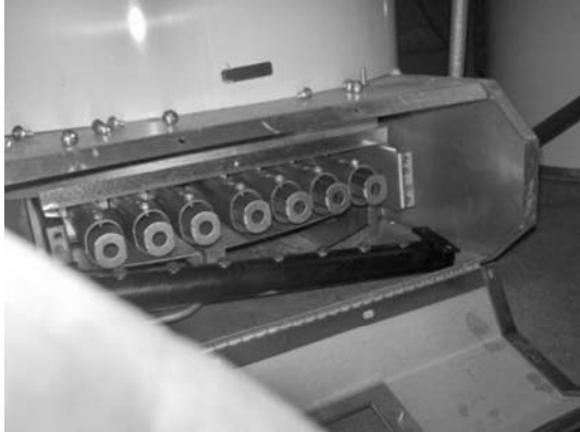
Step 8: Remove manifold from Burners
