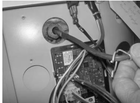
Removing lower sensor from well. Held in place by a clip fastened to well shoulder.
