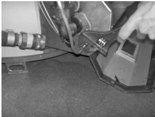
Step 3: Disconnect Pilot Fitting from Burner Box
