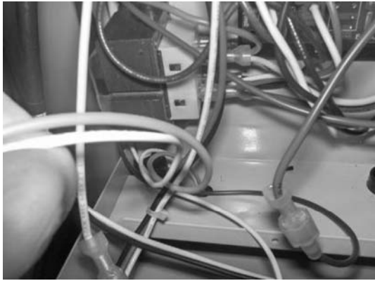
Step 12: Disconnect Pilot wires from control board and remove from Control Box
