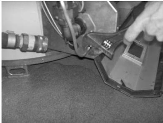
Step 3: Disconnect Pilot Fitting from Burner Box
