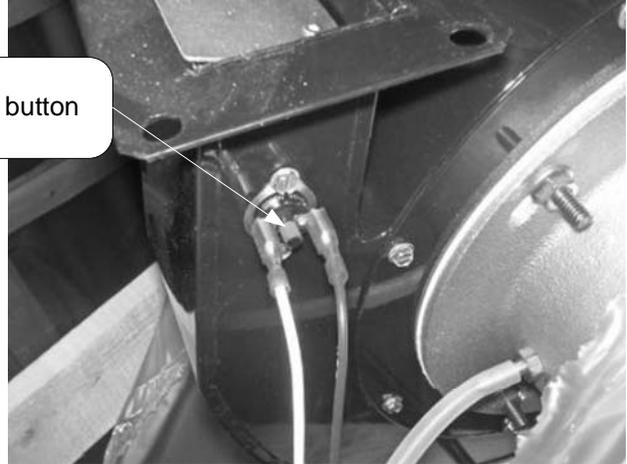
Vent safety thermal switch on PDV-S blower. Depress red reset button in center of switch. If a slight click is felt, switch opened. Check for loose or leaking burner access panel (see section on servicing burners)
