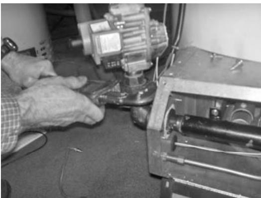
Step 5: Disconnect and Remove Gas Valve
