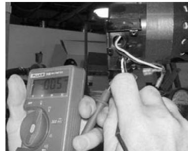
Checking line voltage at the blower wire harness connection on blower.
