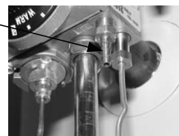
Pressure Tap Shown Installed
