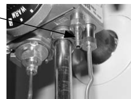
Pressure Tap Shown Installed
