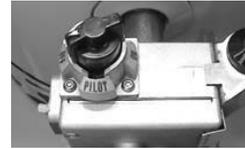
For White Rodgers Control, depress knob slightly and rotate clockwise to the "OFF" position.
