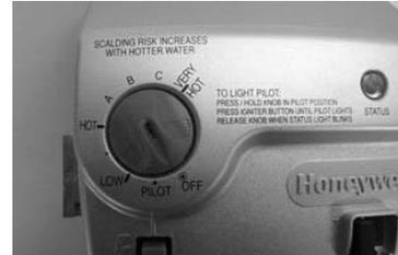
Rotate knob counter-clockwise to the “OFF” position.
