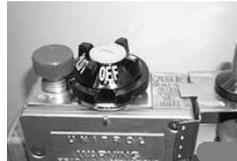
Step 2. Turn off cold water supply to heater. Connect hose to drain spigot of water heater and route to an open drain. Open a nearby hot water faucet to vent heater for draining. Open drain spigot of hot water heater and allow heater to drain to a point below the inlet connection nipple.
