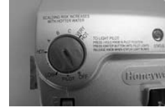
Gas Control shown in the "OFF" position
