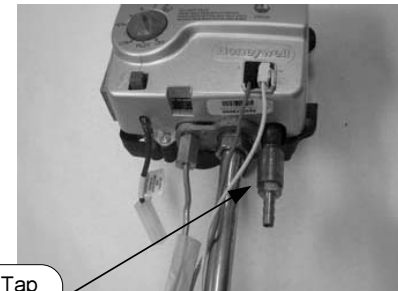
Pressure Tap Shown Installed
