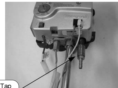
Pressure Tap Shown Installed
