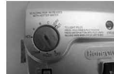
Gas Control shown in the "OFF" position
