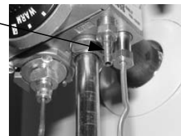
Pressure Tap Shown Installed
