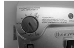
Gas Control shown in the "OFF" position
