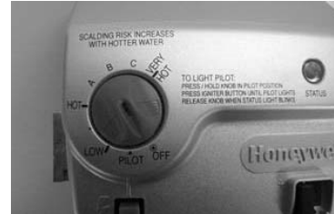
Rotate knob counter-clockwise to the “OFF” position.
