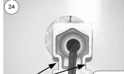
Route wires through relief opening
