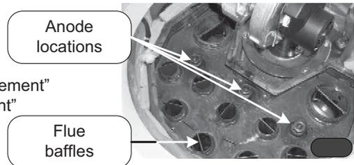
**Note: EF100T399 models have only 1 anode rod under the 2<sup>nd</sup> pass collector cover.**
