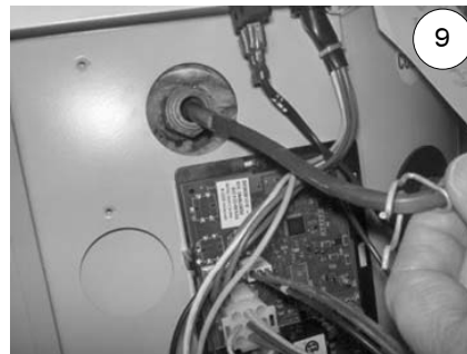
9 Removing lower sensor from well. Held in place by a clip fastened to well shoulder.
