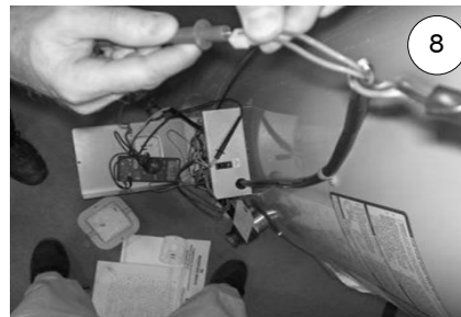
8 Checking continuity of upper sensor wire harness.
